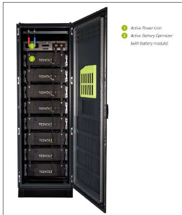
Figure 32: The Battery Management System
