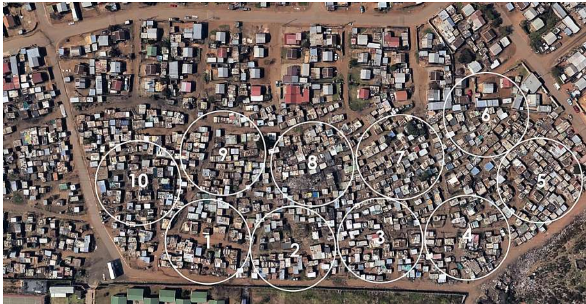
Figure 34: LivPak Sub-Centralised System of 10 dwellings (including School (bottom – green roof) and LivPak Container Hub (bottom middle))
